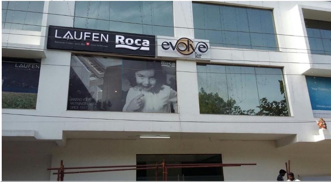
ACP Signage & OWV
